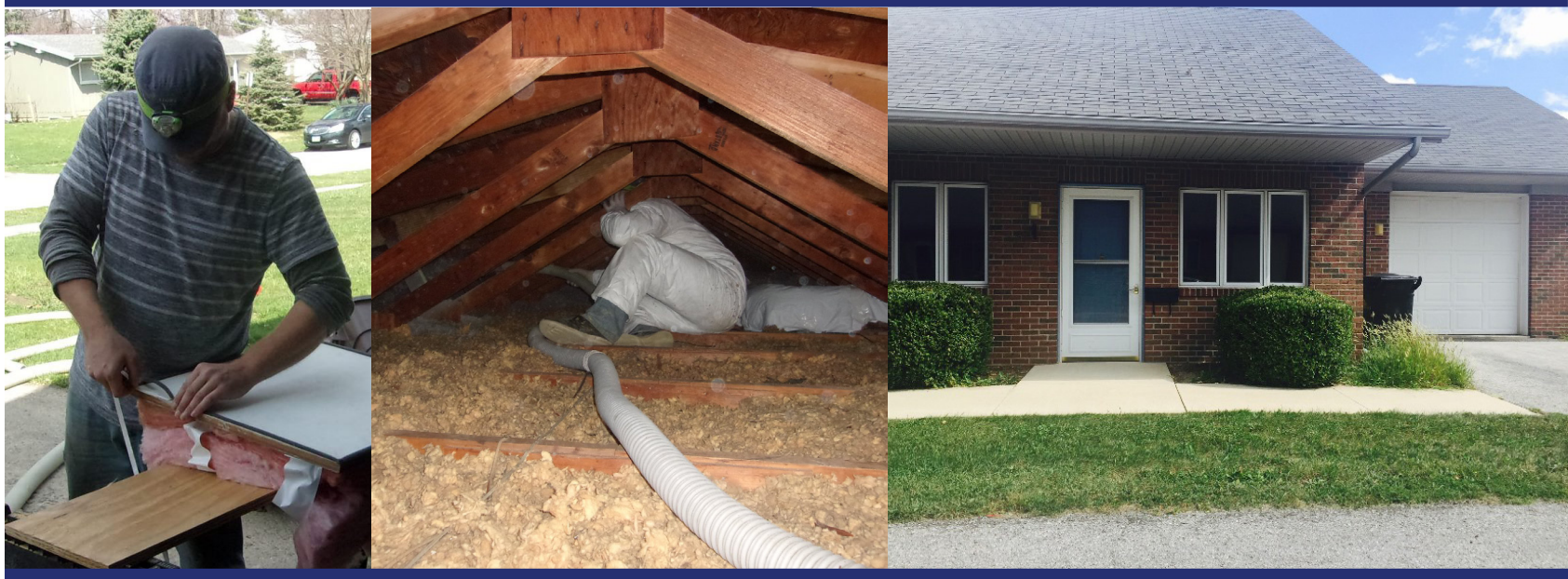
Left photo: Weatherization crew members prep insulation.
