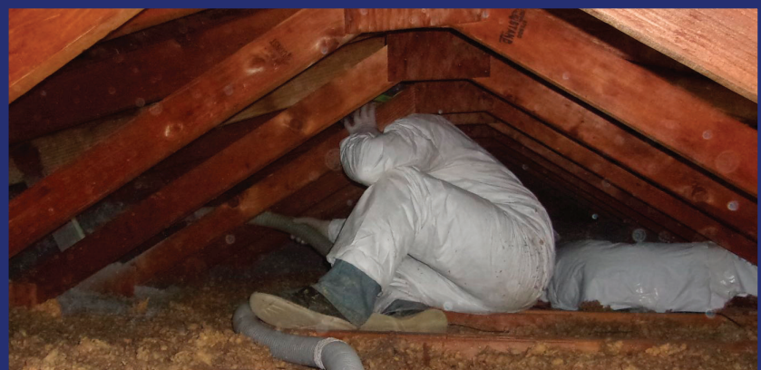
Right Photo: HWAP staff insulates an attic for a low-income home owner
